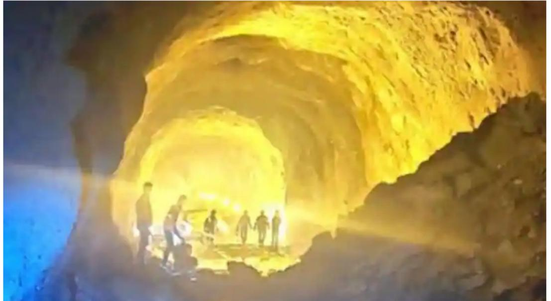
As per the international standards, he said, the escape tunnel constructed parallel to the main tunnel is connected by cross passages at an interval of 375 metres to facilitate rescue and restoration work.
